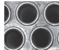
Tube ligaments are .75-inch minimum
